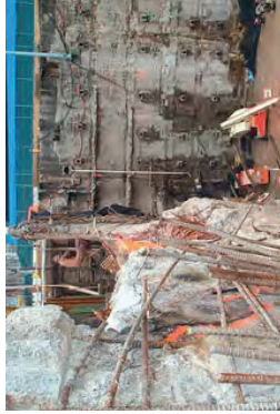
STEP 4: DEMO PORTION OF SLURRY WALL BELOW KEXP
