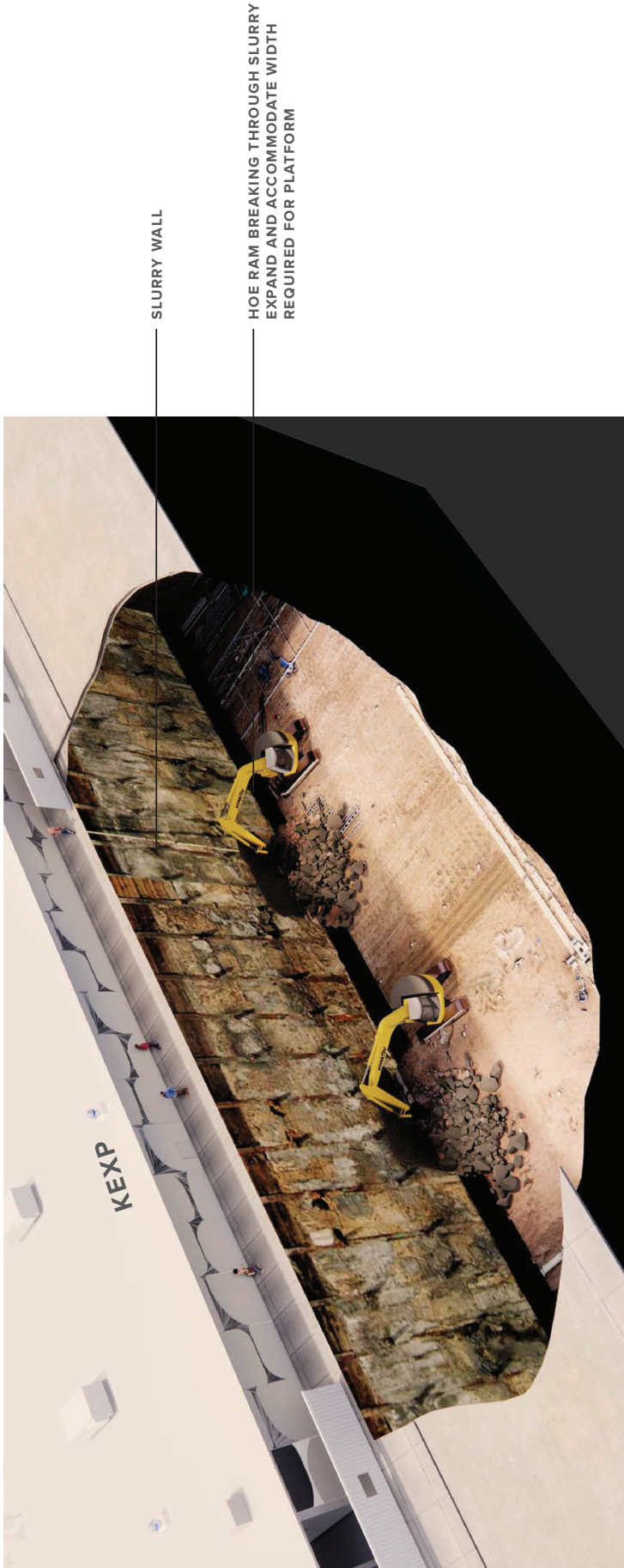
PHASE 4: DEMO PORTION OF SLURRY WALL BELOW KEXP
