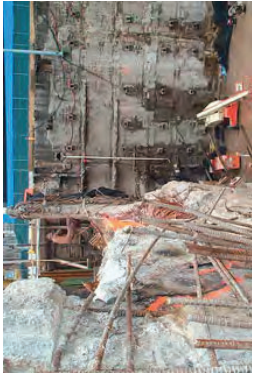
PHASE 4: DEMO PORTION OF SLURRY WALL BELOW KEXP
