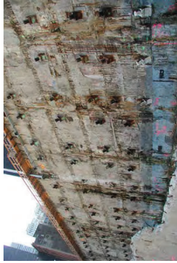
STEP 3: BUILD SLURRY WALL
